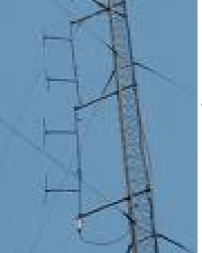
Z<sub>o</sub>= 276 log 2(S/D) S=Distance between and D=diameter
